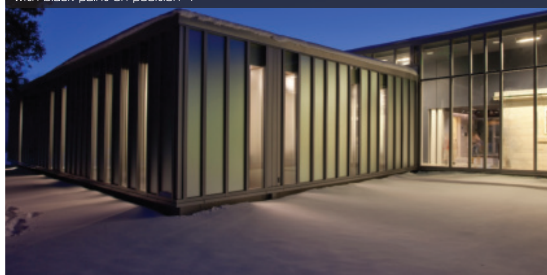
Wellesley College - Wellesley, MA - 6mm clear glass Satin on position 1 with black paint on position 4
