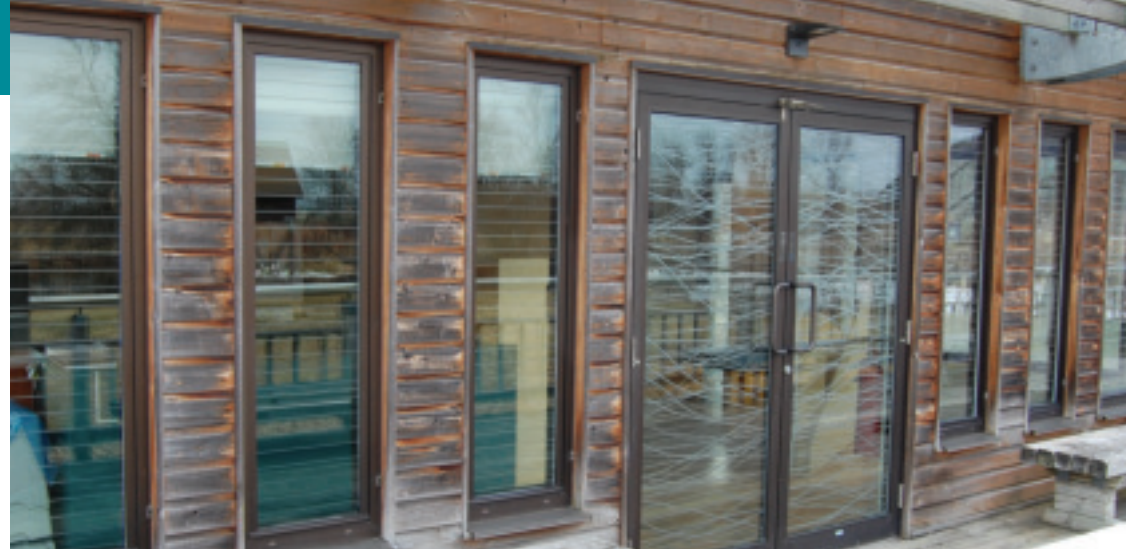
Bird Friendly Project - Cap Tourmente National Wildlife Area, St-Joachim, QC AviProtek patterns 213 and 214 on position 1
