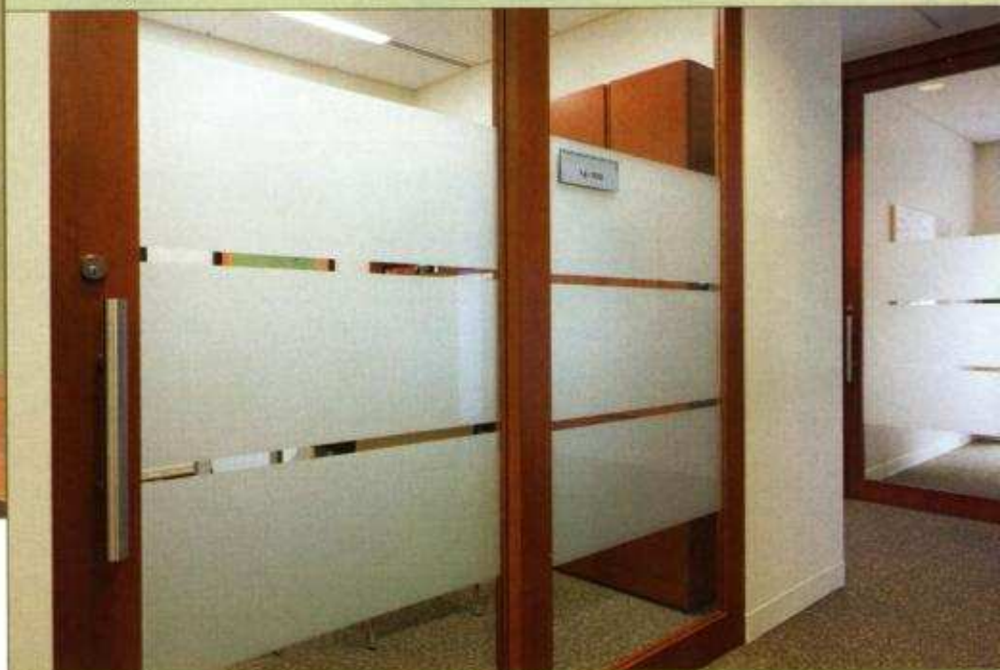
Acid-etched glass can be used for interior office applications, such as Moody's Investor Services in New York City, providing aesthetics as well as privacy.
